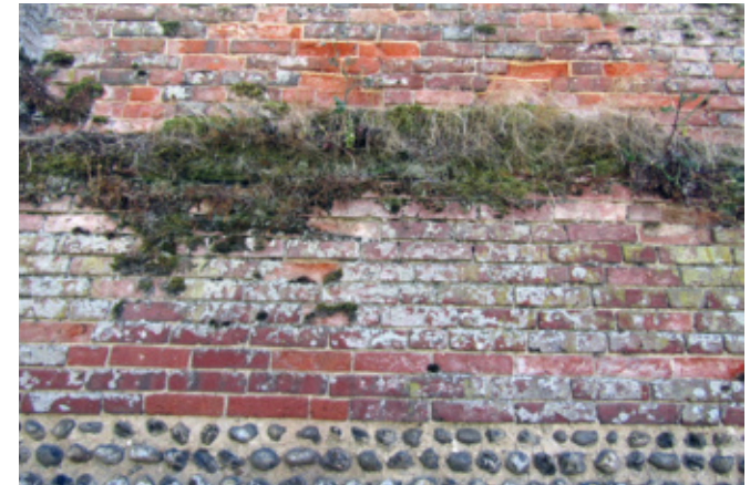
Vegetation growth to a wall
