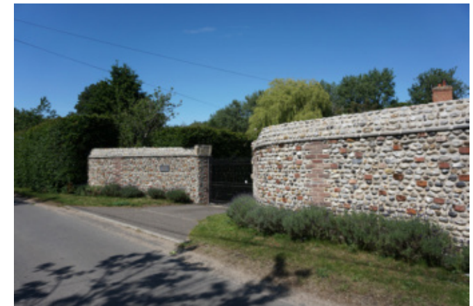
New walls and gate at Green Farm
