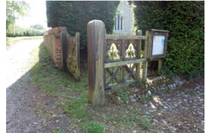
View of the churchyard wall showing a decorative wooden and iron gate
