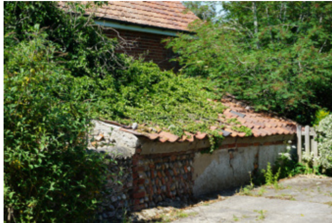
Outbuilding in poor condition with overgrown vegetation
