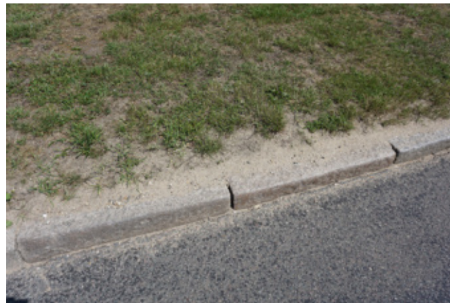
Granite kerb stones on Hunworth Road
