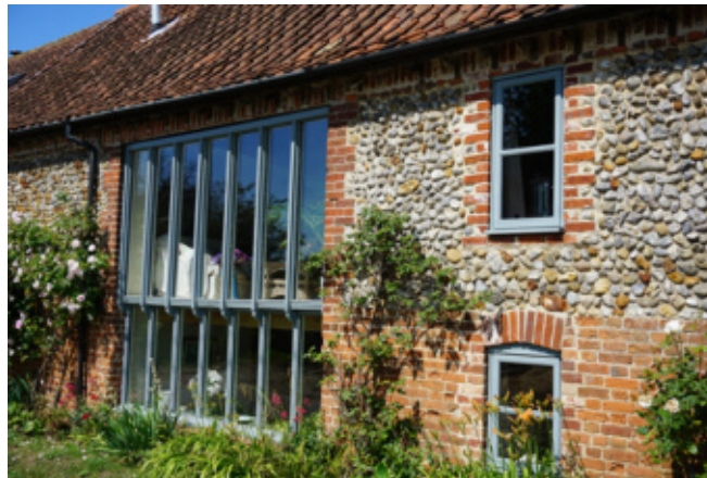
A sensitive barn conversion on King Street
