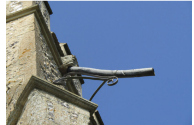
Detail of a gargoyle on west tower
