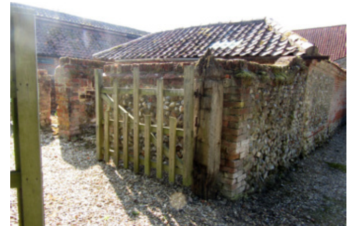
Former pigsties at Hunworth Hall Farm
