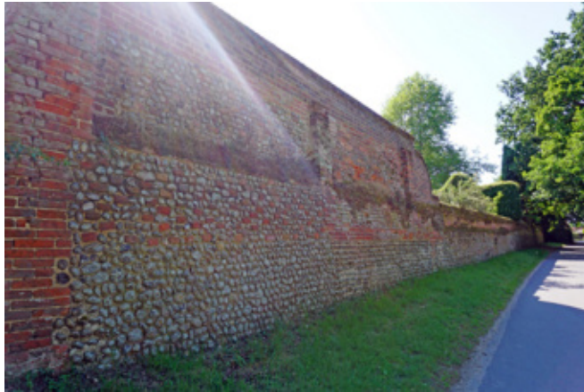
Boundary wall to Hunworth Hall
